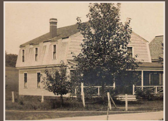
Blake House in East Sebago, original home of the Baldwin & Sebago Telephone Company
